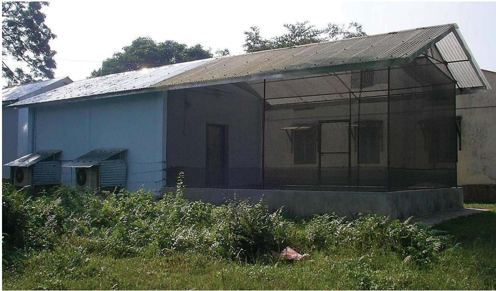
Fig. 10.5. The purpose-built rust propagation facility at Assam Agricultural University. Plants were maintained in the net house (right) and inoculated in the air-conditioned mist chamber (attached to left of the net house). The control room for the facility is in a separate building situated to the left of the mist chamber. Photo courtesy C.A. Ellison.
